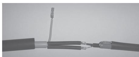
8. The two heating cable conductors are connected with the two 1.5 mm<sup>2</sup> rivets of the two cold tail conductors (L+N).
