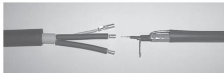
7. Crimp tube 4/1, L=45 mm is pulled in over the two conductors (L+N) of the cold tail.
