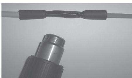
14. Crimp tube 12/3, L=150 mm is pulled over the entire connection. The crimp tube is crimped down from the middle out towards the ends.
