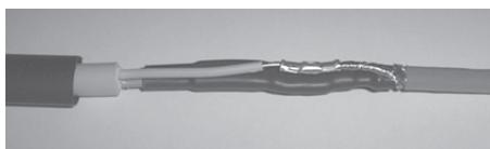
13. The heating cable screen is connected with the 2.5 mm<sup>2</sup> rivet on the cold tail screen/ground wire. The rivet is squeezed onto it.
