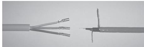
6. Now the two cables are ready for assembly. 1.5 mm<sup>2</sup> rivet is squeezed onto the two conductors (L+N) and 2.5 mm<sup>2</sup> rivet is squeezed onto screen/ground wire, all on the cold tail.
