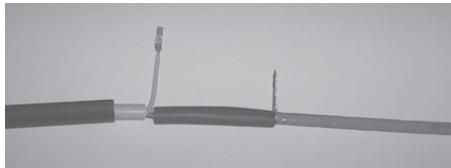
11. Crimp tube 9/3, L=85 mm is pulled over the connection to ensure that the screen/ground wire is still free.
