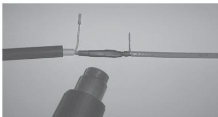
12. The crimp tube is crimped down from the middle out towards the ends.
